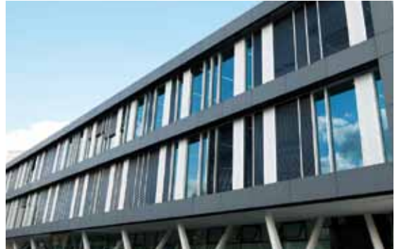
Technology & Innovation Center at the Meitingen site
